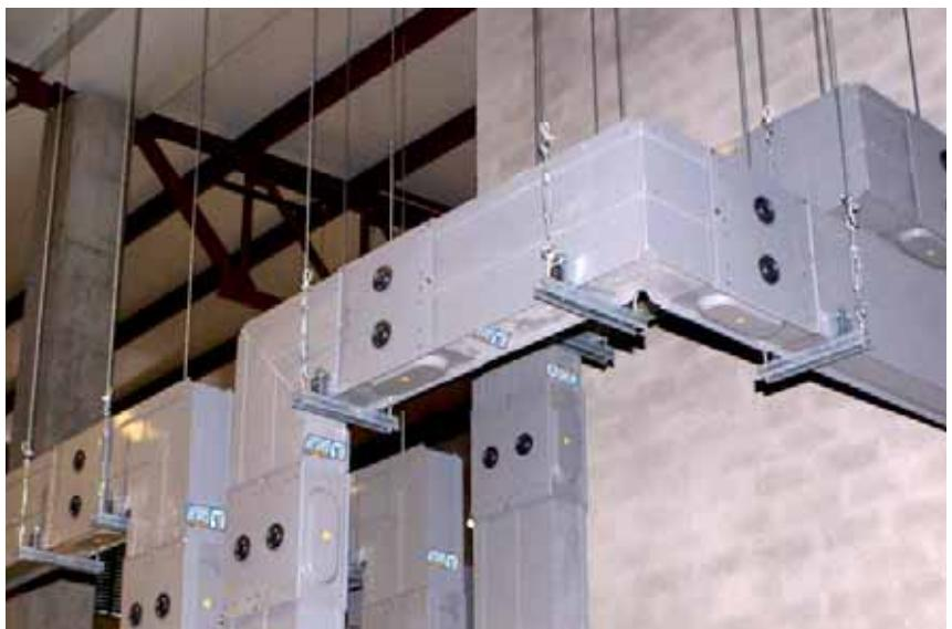
The IMPACT busbar trunking system is designed for power transport and distribution and is especially suitable in the electrical switchroom both as a transformer-switchboard or switchboard-switchboard connection and as the main power distribution system for industrial, commercial and service industry.
